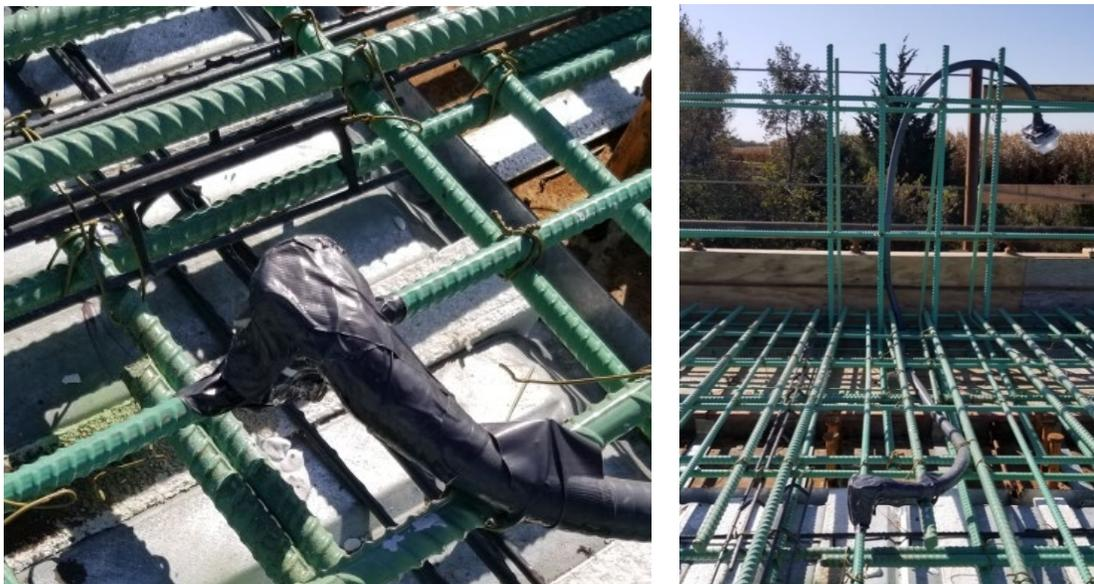
**Figure 39.** Valparaíso Bridge Instrumentation: (a) gypsum seat attachment of the ultrasonic transmitter wrapped in duct tape; (b) Sensor cable is protected inside a protective duct and ran to the side of the bridge
