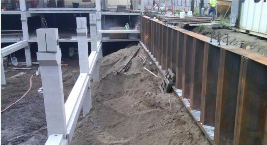
Figure 2.13 An example of sheet piling as a permanent foundation (with a temporary soil berm) for the construction of below-grade precast concrete framing (Underwood, 2020).
