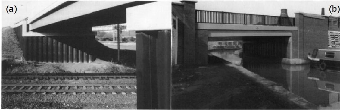
Figure 1.5 An example of sheet pile abutment bridges in Europe. (a) Humber Road bridge (Immingham, UK), and (b) Canal bridge (Stoke-on-Trent, UK). Images are from Yandzio (1998).
