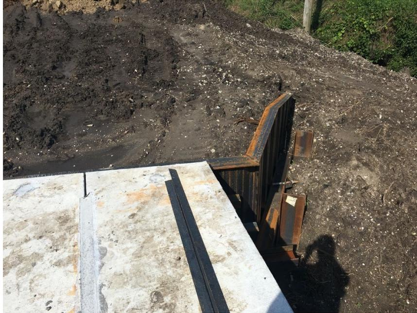
Figure 1.6 An example of a county bridge in Nebraska with solid planks and sheet pile abutments.
