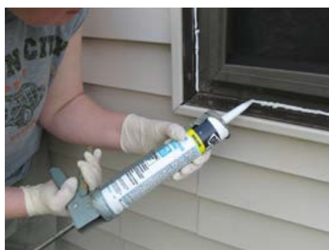
Caulk cracks around windows.
