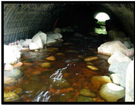
Figure 1. Example of the inside of a stream simulation (SS)-design culvert (1a) and a bankfull and backwater (BB)-design culvert (1b). The SS-design example on the left (1a) shows how substrate is used to construct banks within the culvert so that the fish does not know the difference from the adjacent stream channel. The BB-design example on the right (1b) does not have constructed substrate within the culvert [Colour figure can be viewed at wileyonlinelibrary.com ]
