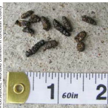
Bat scat (guano) can be found in porches, under eaves, and other places bats hang out.
