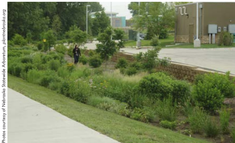
Fireworks restaurant bioswale in Lincoln captures stormwater from adjacent parking lots and buildings absorbing excess runoff, filtering pollutants and creating habitat for birds and insects. This project completely changed people's experience along this part of Antelope Bike Trail, acting as a catalyst for continued greenspace improvements along the trail.
