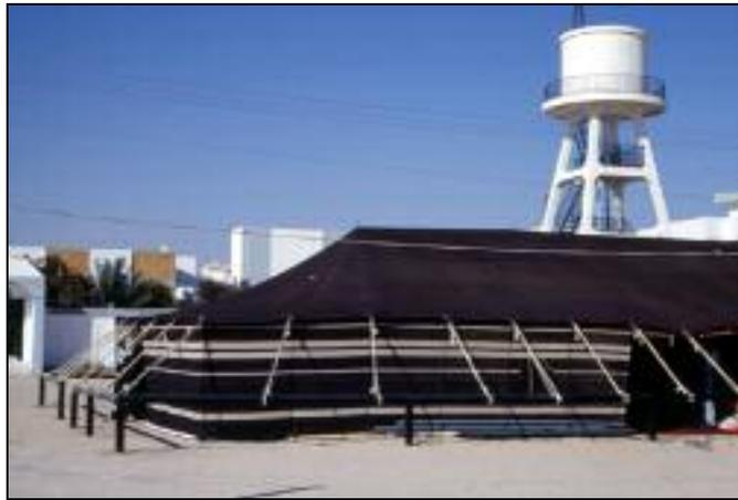
*Fig. 5. A new tent in the same location in Haneedh. Note the same water tower. Instead of long tensioning ropes, the tent is supported by metal poles inside and posts outside, with short tensioning ropes. 1993.*
