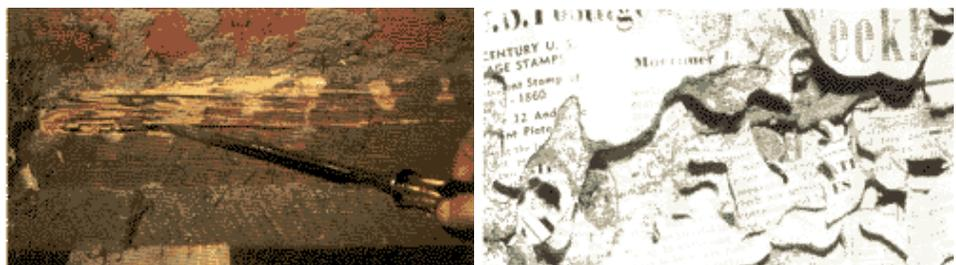
**Figure 1. Termite Damage.**
