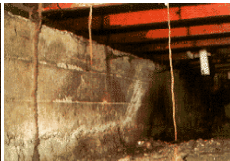
Figure 4. Termite infested wood and mud tubes.
