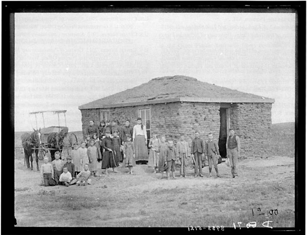
Students and teachers in front of sod schoolhouse, Custer County, Nebraska. 1891. Solomon Butcher photograph, Nebraska State Historical Society. Reprinted by permission.
