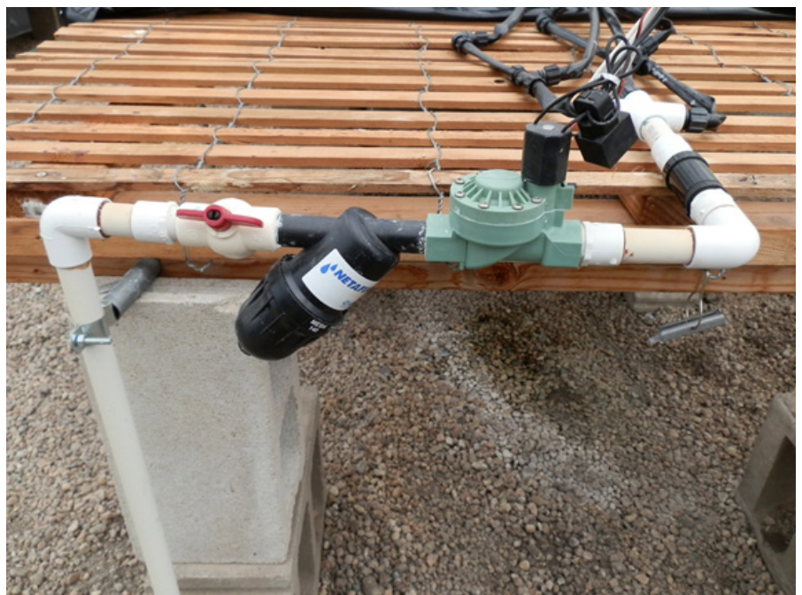
Figure 12. Irrigation supply to individual bench includes manual shut off, 140 micron mesh screen filter, 24 volt solenoid valve, and 10 psi pressure reduction valve prior to the Capmat II distribution manifold.
