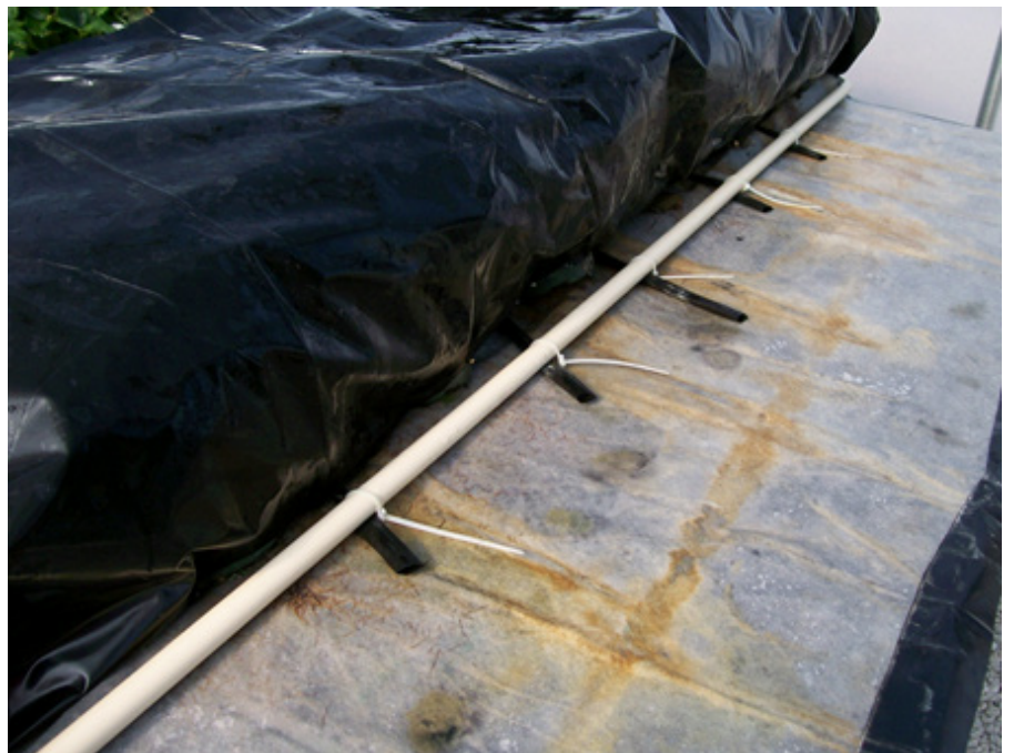
Figure 6. Ends of seep hoses are wire tied to 3/4-inch PVC pipe to maintain spacing between each length.
