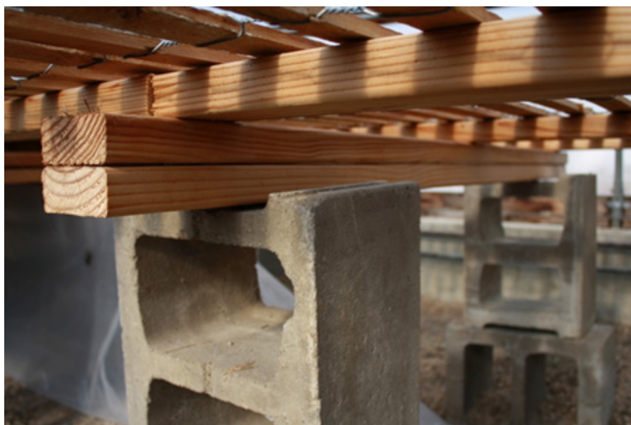
Figure 2. Cross-arm positioning with bench top support members and woven bench fabric installed.
