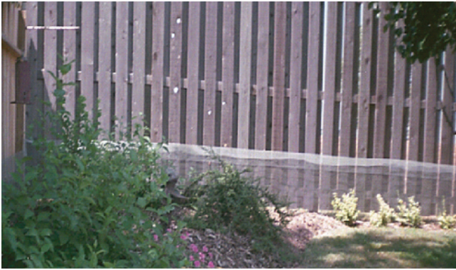
Figure 4. A rabbit fence added to an existing fence.
