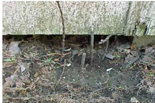
Figure 2. Hole entrance with twigs in front to test for animal use.
