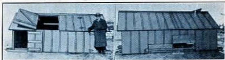
FIG. 10.—Front view of the two-sow "blizzard beater" showing doors open and closed, and back view of the same house showing the ventilators
