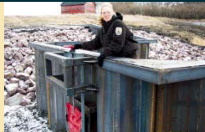
Katie Goodwin, refuge operations specialist at the Morris Wetland Management District, Minn., shows the recently completed box weir on the Centennial WPA. (USFWS photo)
