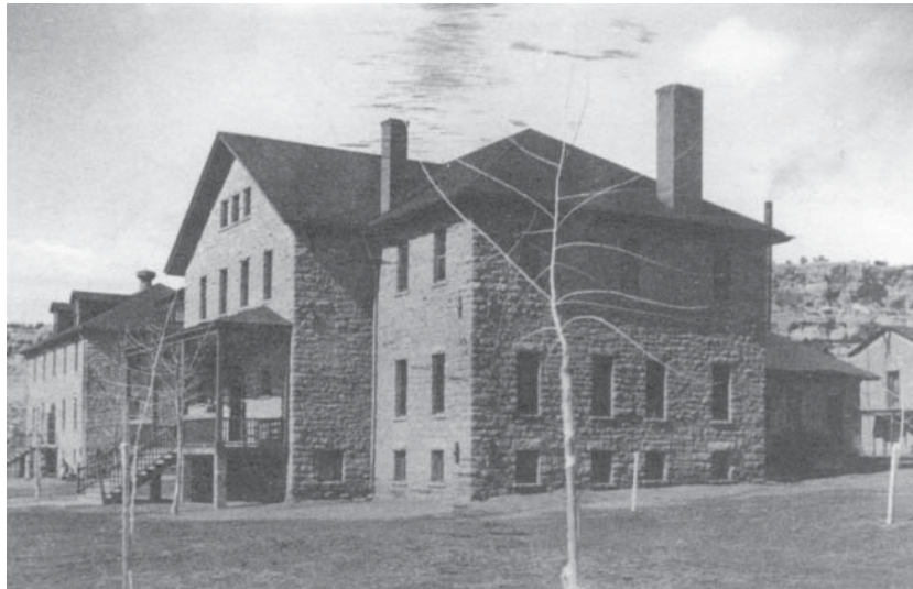
Keams Canyon school building. (AHS/SAD MS 1195)
