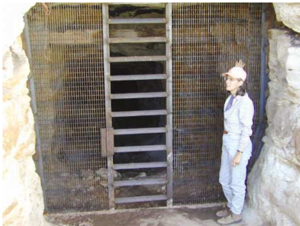
Figure 1. A typical bat gate.
