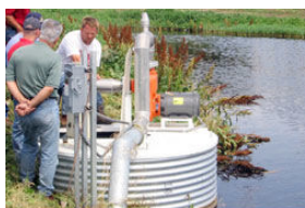
A pump used to move runoff from a small debris basin to a vegetative treatment area.
