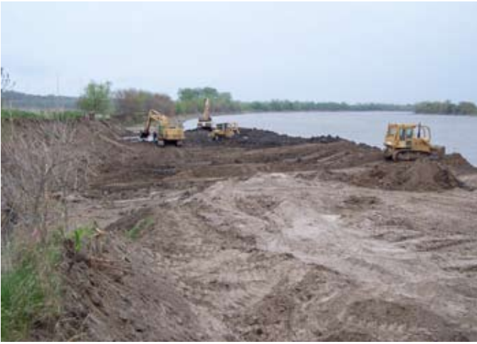
Constructing shallow-water habitat on the Missouri River.
