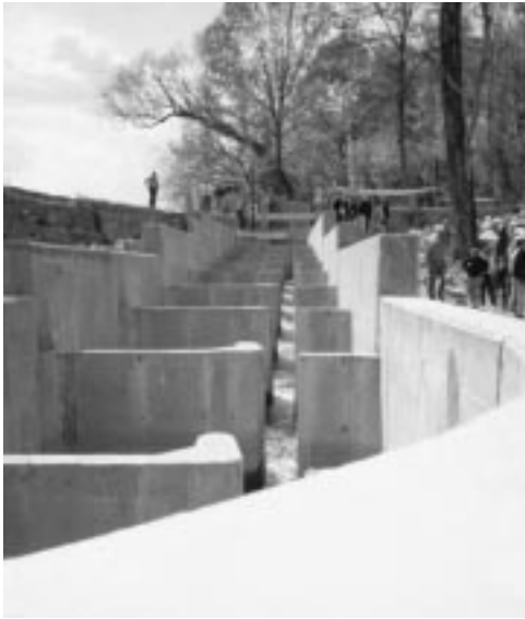
Safer for shad. A fishway at Boshier Dam in Richmond opens another 138 miles of the James River to the American shad, once Virginia's most bountiful fish. "Our best times are ahead," said Virginia Lt. Gov. John Hager at the April 21 dedication. Photo by Ken Burton.
