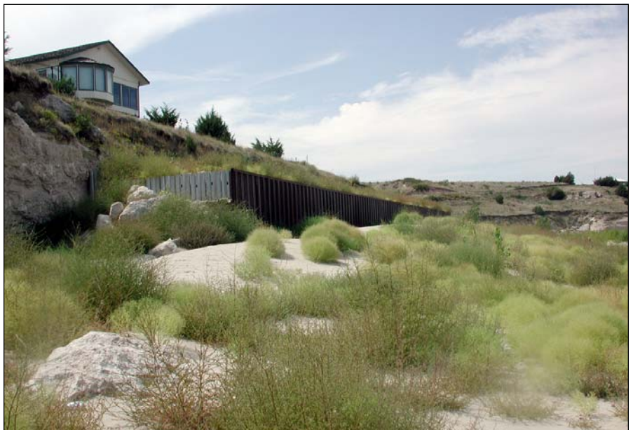
A seawall helps protect residential property from erosion damage on the southeast shore of Lake McConaughy north of Ogallala, Neb. Continued drought has shrunk the state's largest reservoir and revealed previously unseen effects of more than 60 years of shoreline erosion. Some property owners have built seawalls or graded cliff faces to slow erosion. University of Nebraska-Lincoln geologists are studying the erosion to learn more about its impacts in reservoirs. (NU Institute of Agriculture and Natural Resources photo.)
