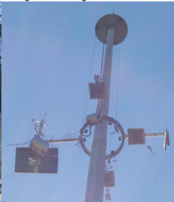
Figure 4. Raising the LLWAS Remote Station
