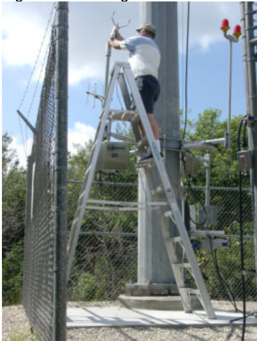
Figure 3. Installing the Sonic Sensor
