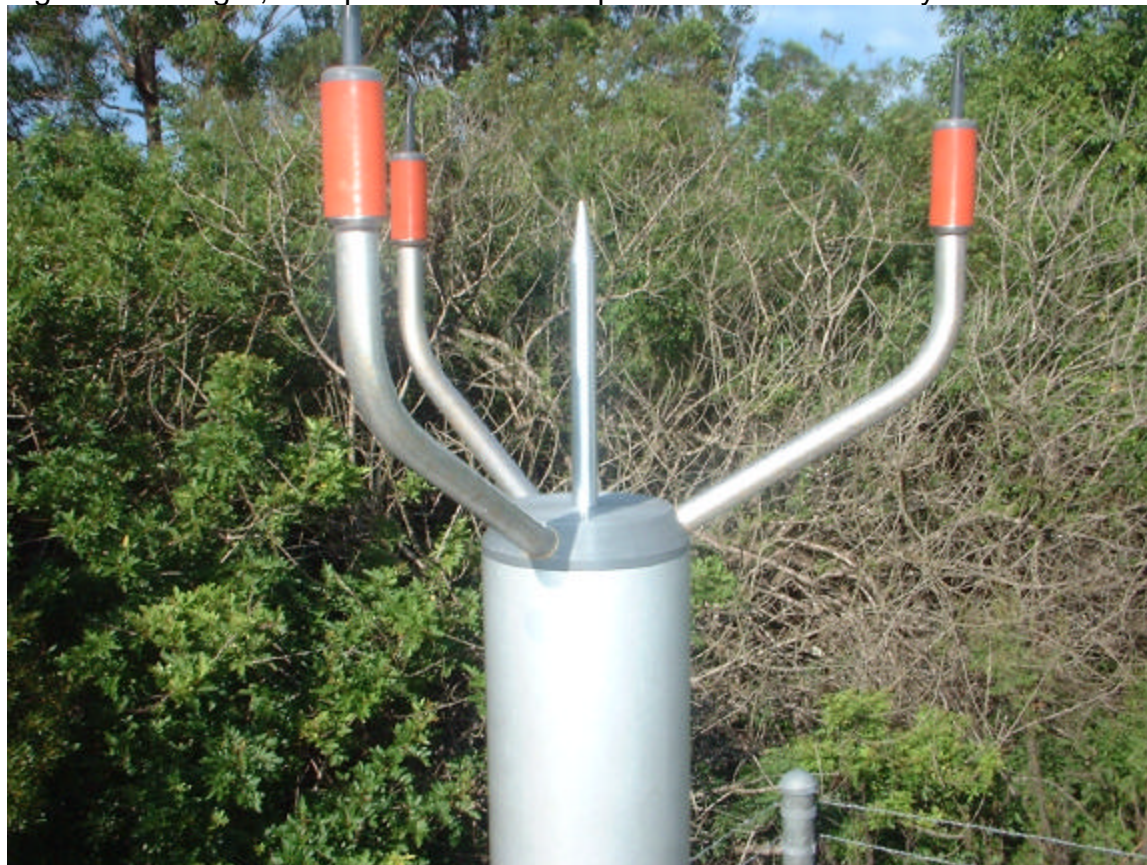
Figure 13. Longer, Sharper Central Bird Spike Installed at Fort Myers
