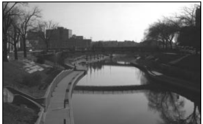
A stretch of Kansas City's Brush Creek flood control and transportation corridor near the Country Club Plaza area. The project has been under development since 1978 and bears similarities to Lincoln's proposed Antelope Valley project (photo: Steve Ress).
