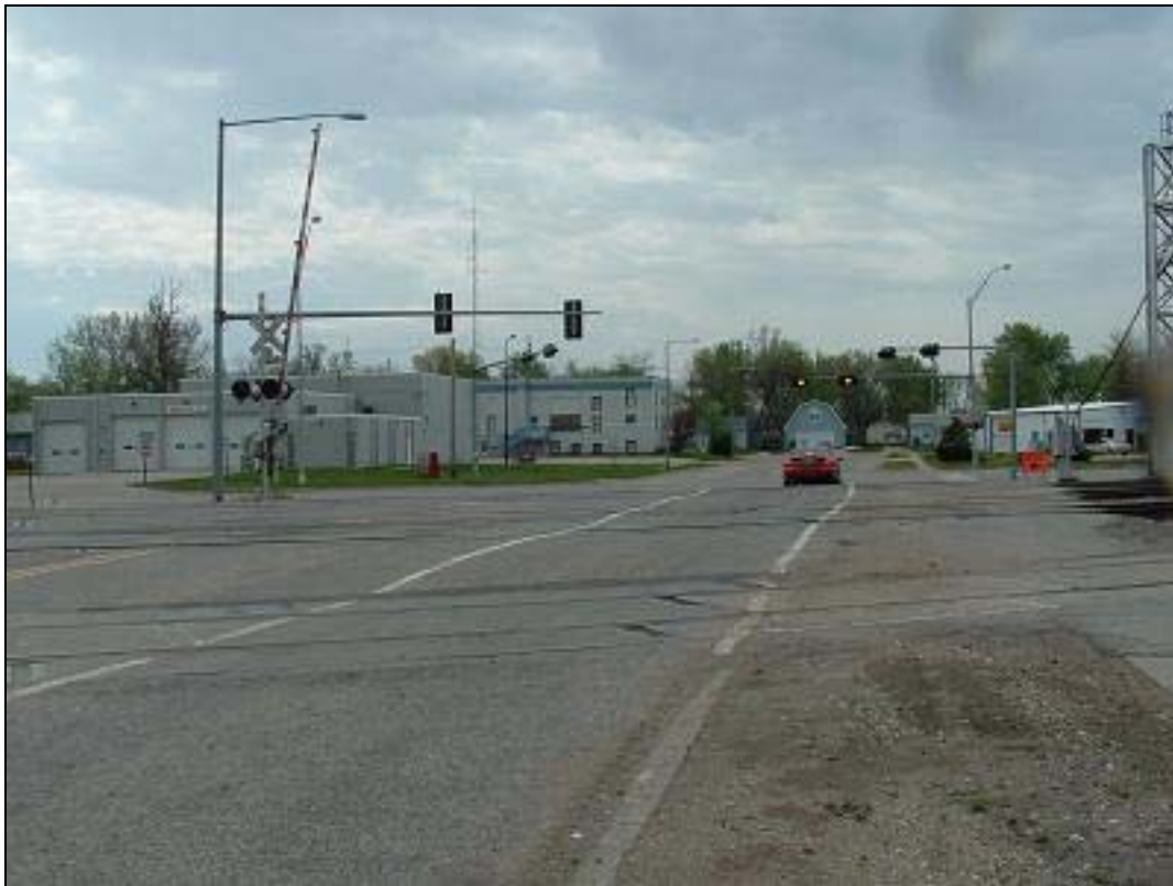
Figure 3.1. Grade crossing at North 141 st Street in Waverly, NE
