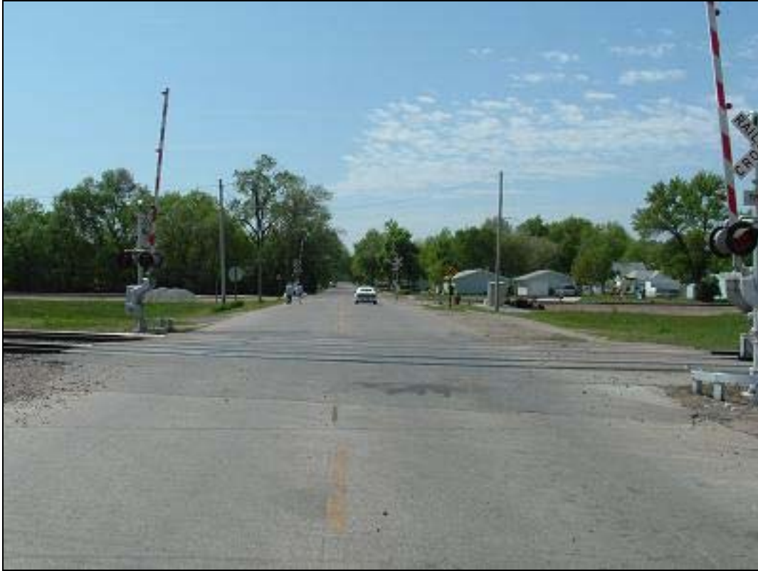
Figure 3.2. Grade crossing at M Street in Fremont, NE
