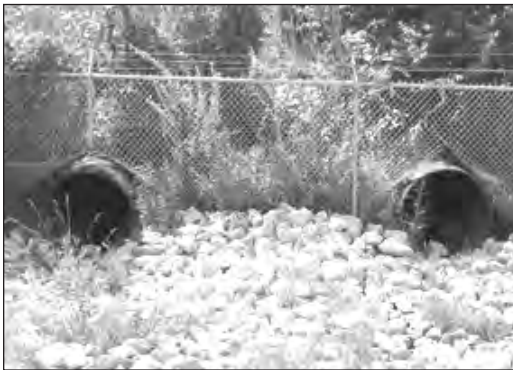
FIGURE 1. Culverts through a fence line can create large passageways for wildlife at airports. (Photo by J. E. Kubel)
