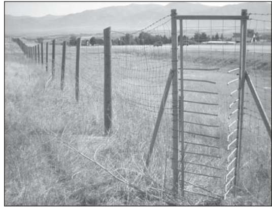
FIGURE 1: One-way gates allow deer to exit the roadway should they become trapped within the fencing.
