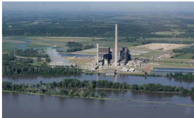
This power plant near Nebraska City was nearly underwater from Missouri River floodwaters in June. The Water Center's annual water and natural resources tour will explore effects from the flood and lessons learned this coming July.
