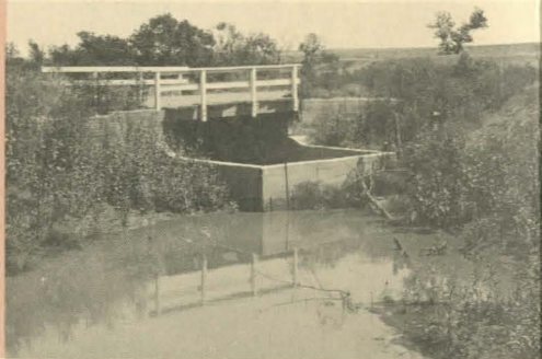
Gully control with the proper county road structure.
