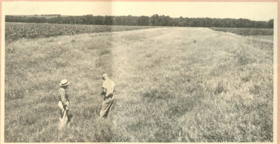
5. Level gully and seed it to the proper grasses.
