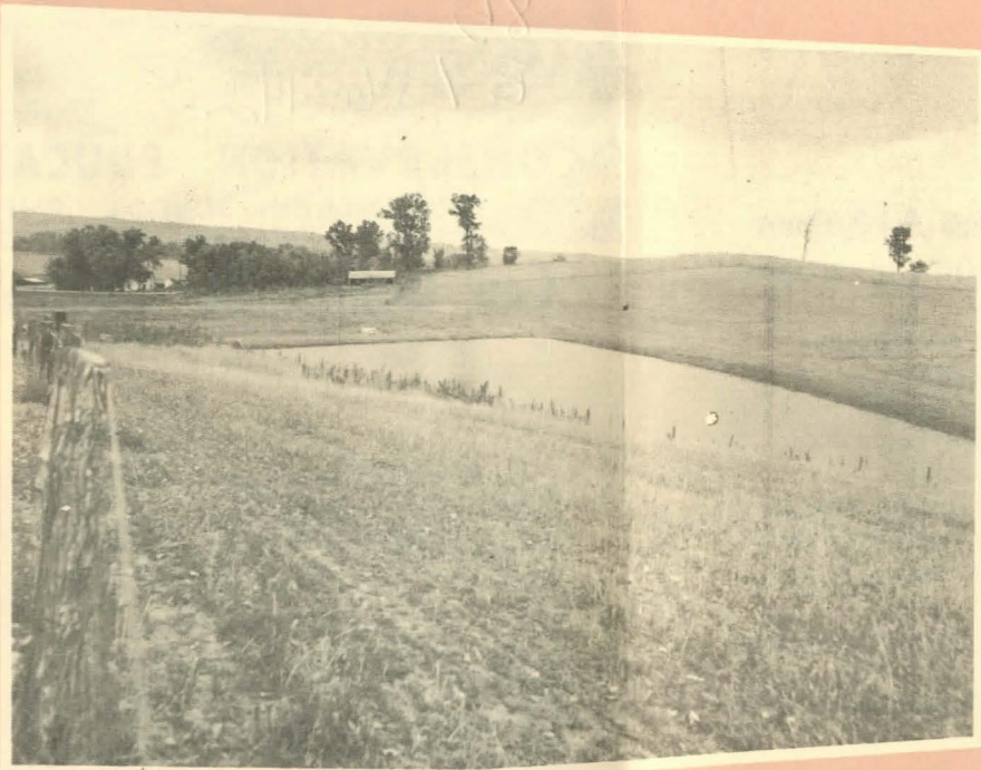
2. Build an erosion control dam.
