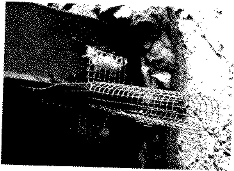
Figure 5. The Hanks' excluder device is a hardware cloth oval cylinder that extends the opening of the roost away from the building. The dimensions of the device are dictated by the species of bat being evicted.
