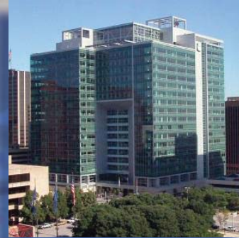
Union Pacific Headquarters Building
